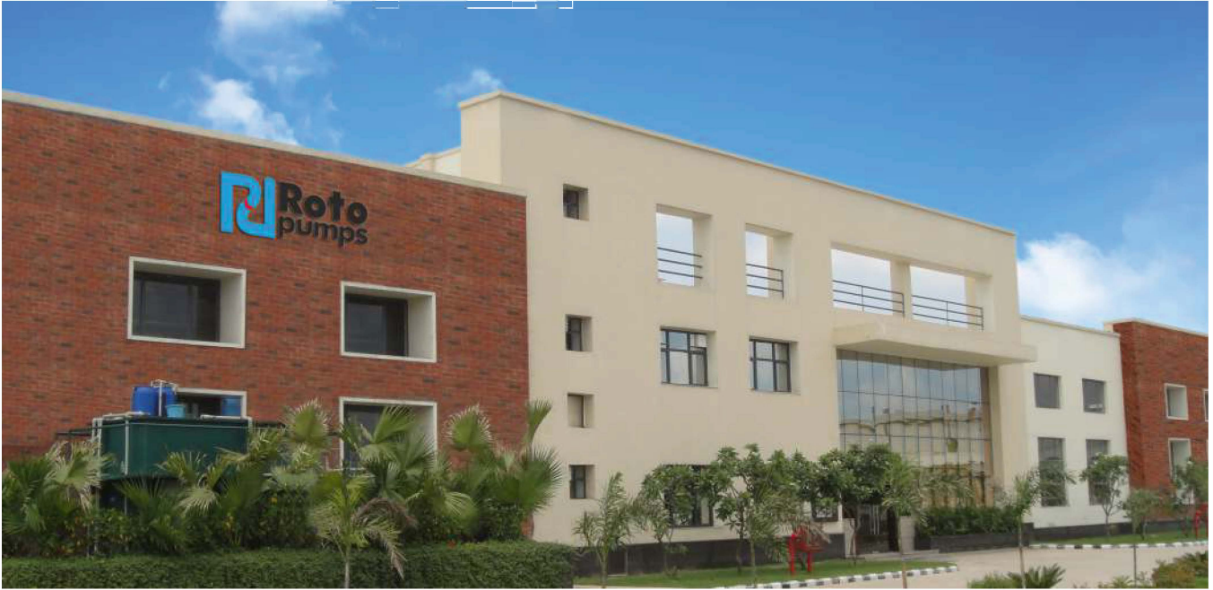
Roto Pumps Limited, Manufacturing Plant, India
