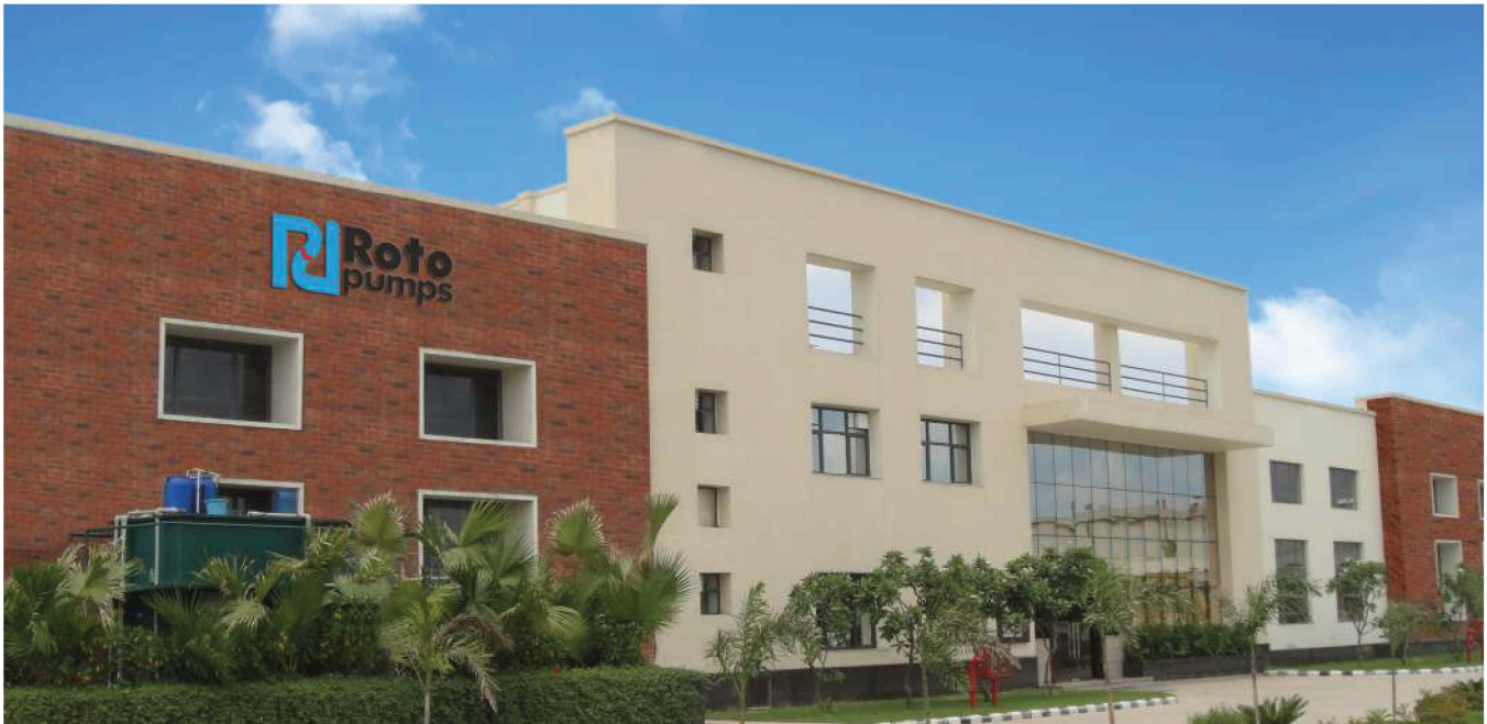
Roto Pumps Limited, Manufacturing Plant, India
